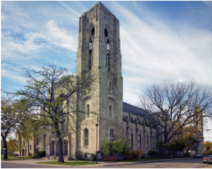
AltusWorks performed an extensive Facilities Analysis of the First Presbyterian Church complex in Chicago, IL.
