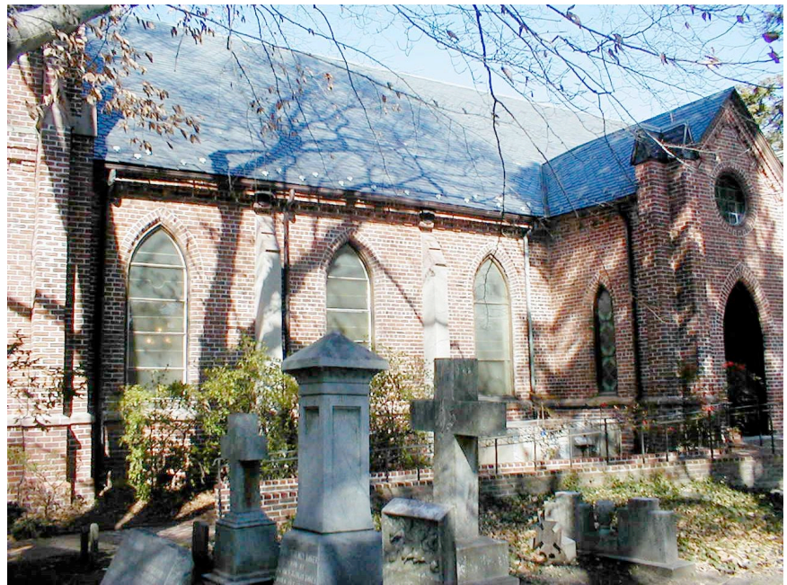
Calvary's congregation installed brick ramps (in background) complimentary to the design of the Gothic church to make the building accessible.
