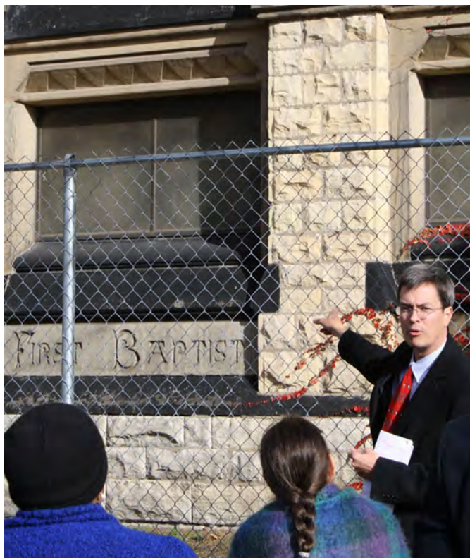
Architect and Advisory Board member Nevin Hedlund, sponsor of an interfaith New Dollars/New Partners training that is taking place in Chicago, explains masonry care and maintenance to participants at Olivet Baptist Church (formerly known as First Baptist).
