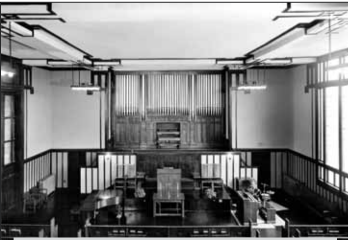
Redeemer Missionary Baptist Church, Minneapolis. Full renovation of this historic Prairie School church included meticulous restoration of original details and the discreet introduction of new amenities such as a baptismal pool in the sanctuary. (Can you spot it?) The project received an Honor Award from the National Trust for Historic Preservation.
