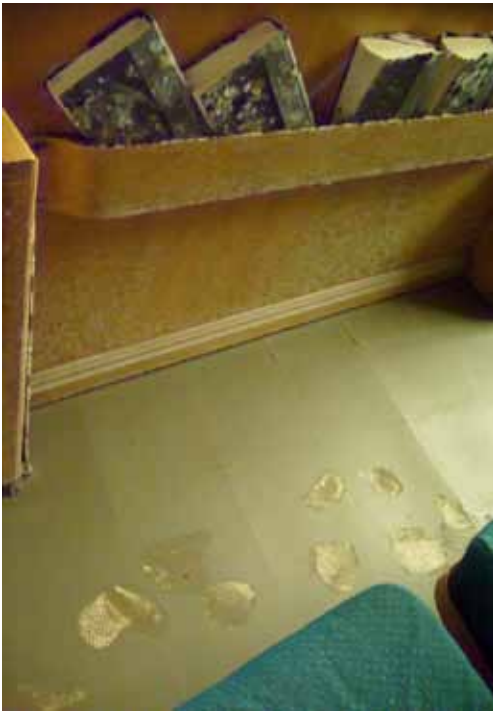
Photos of Congregation Beth Jacob in Galveston, TX, show the damage caused by Hurricane Ike. Silt and mud covered the floors and walls; surging water damaged furniture and textiles. Photos courtesy of Congregation Beth Jacob.
